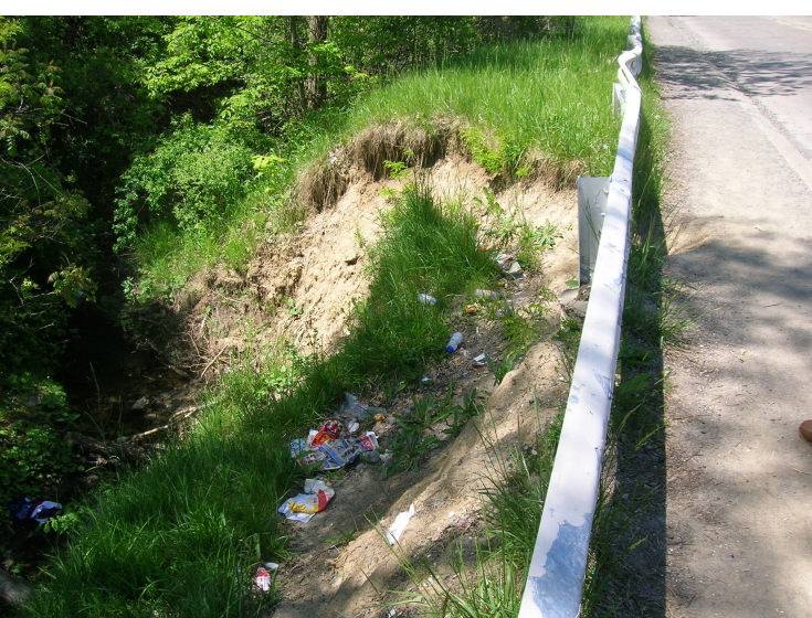
High water velocities are clearly significant and causing massive erosion
