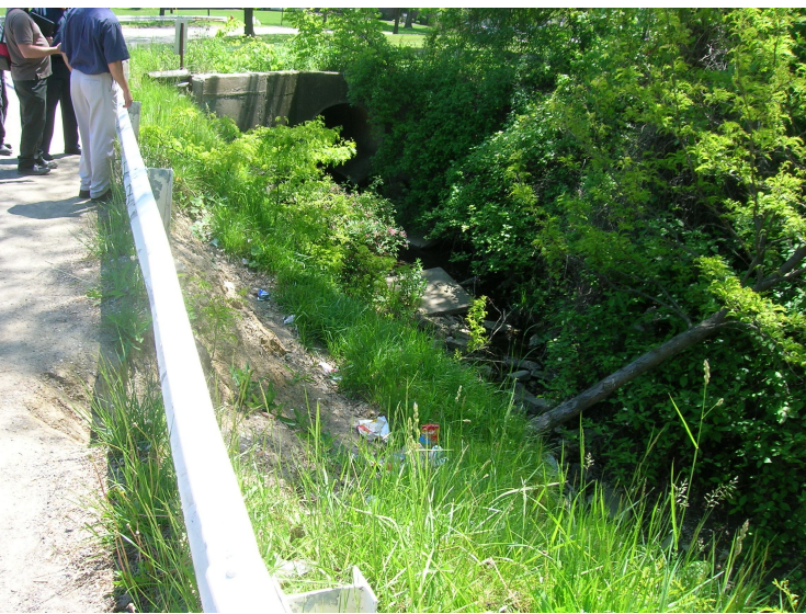
Bear Creek eroding, channelized, and jeopardizing the integrity of the road due to increased storm water runoff
