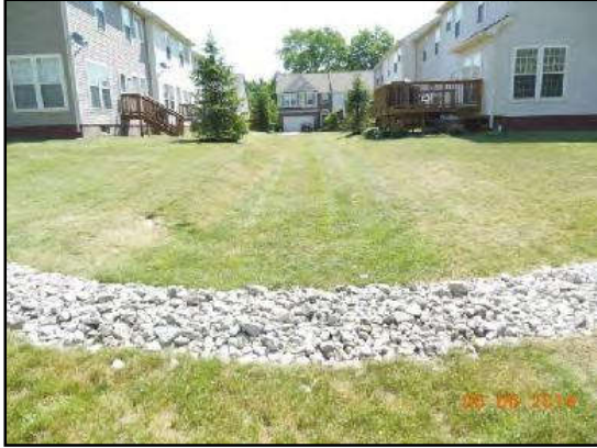
Well maintained vegetated infiltration swale with stone check dam. Credit: Chagrin River Watershed Partners, Inc.
