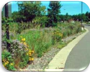
Curbside street with infiltration strip in MN
