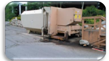
Dumpster leaking directly into a storm sewer
