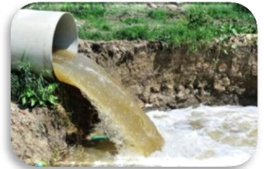
Stormwater outfall in Baltimore County, MD
