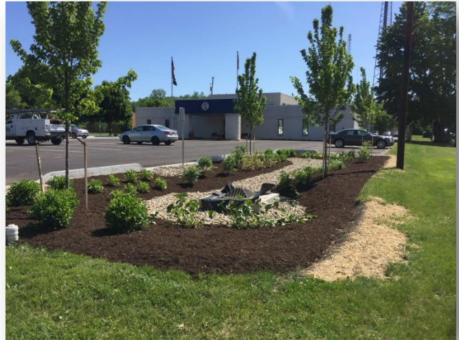
Bioretention cells retrofit in Madison Township, OH
