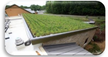
Green roof at West Creek Reservation's Watershed Stewardship Center in Parma, OH
