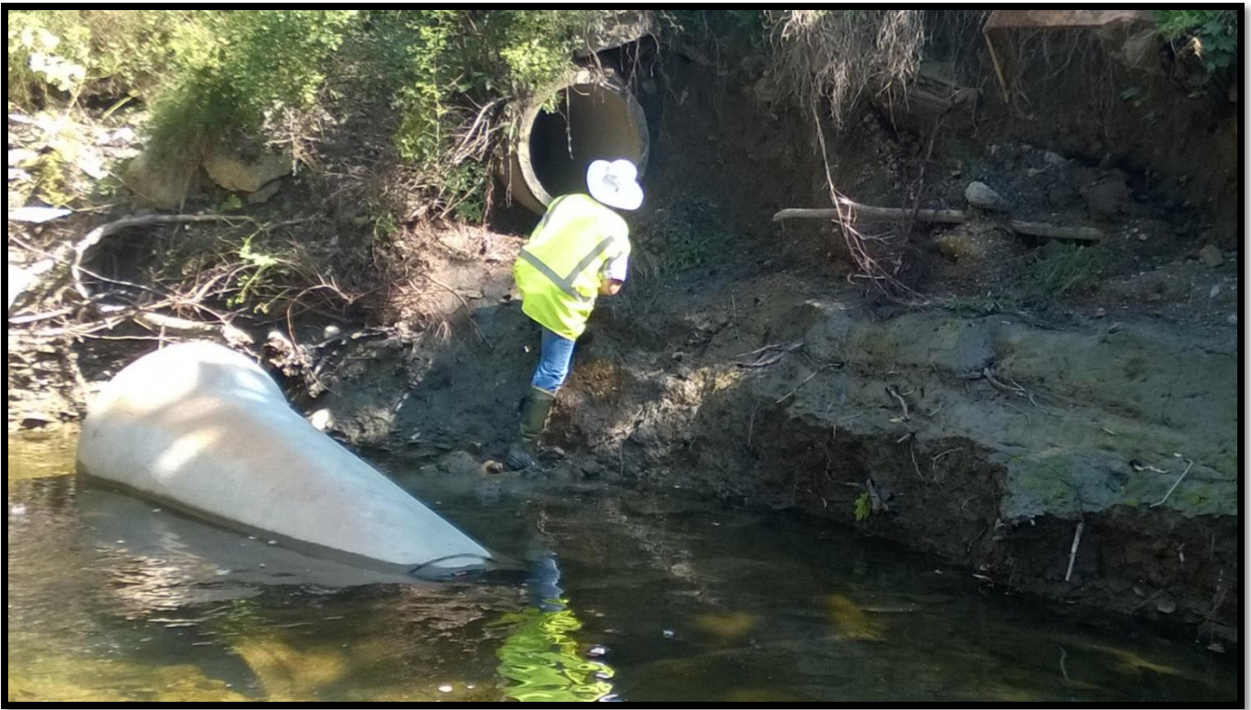
Figure 15: Bear Creek, Town of Twinsburg HUC-12, showing in-stream erosion at culvert
